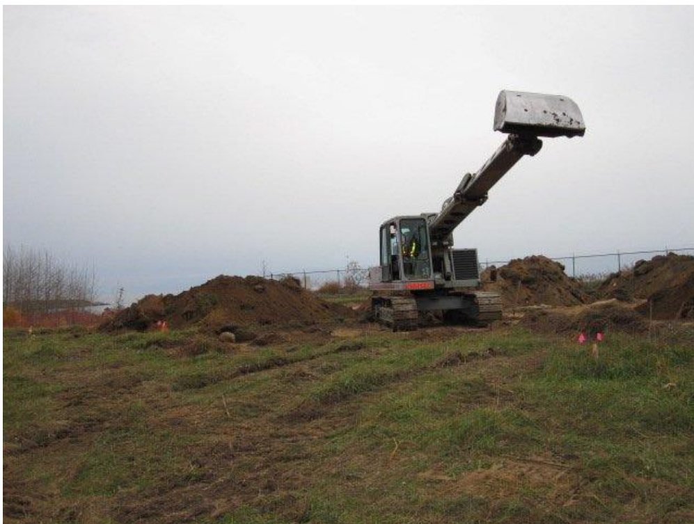
Plate 2: Gradall stripping at the Brady site (ALGq-83), looking southeast.
